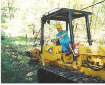
Equipment Operator Frank Arch plows in the new underground primary conductor in the Chequamegon National Forest.
